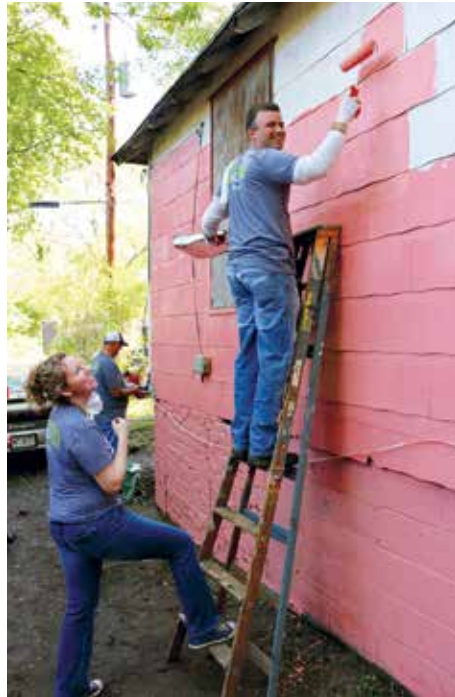
ALPHARETTA EMPLOYEES PAINTING A HOUSE'S EXTERIOR
